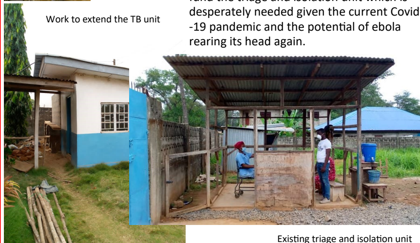
Existing triage and isolation unit
