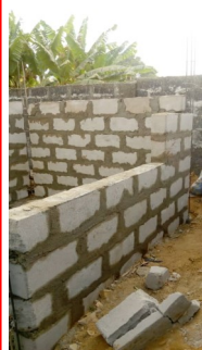
Work to extend the TB unit
